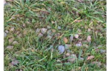
parking terre-pierre enherbé
